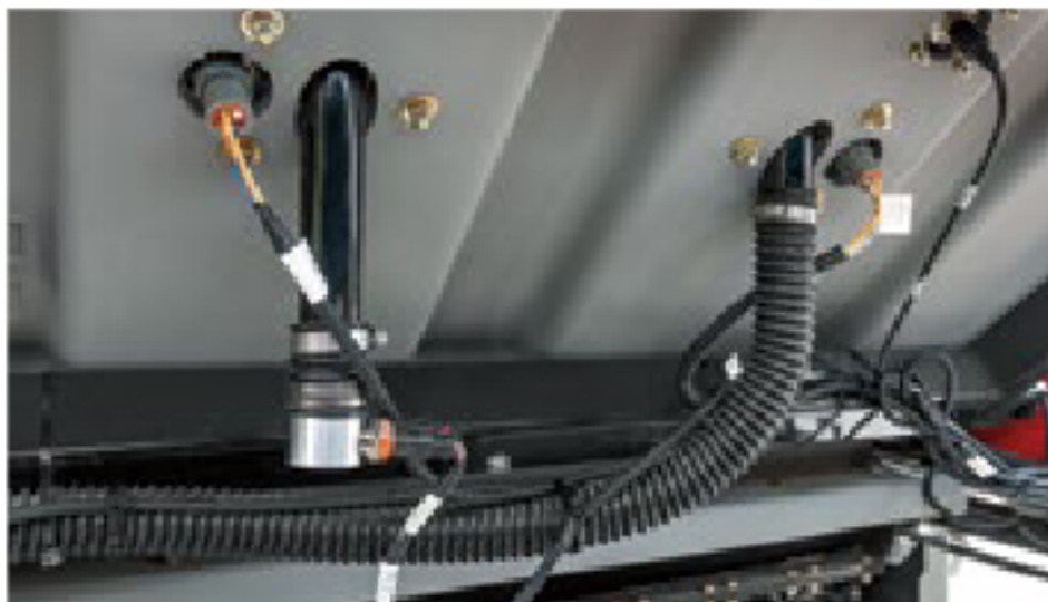
Tank pressure sensors.
